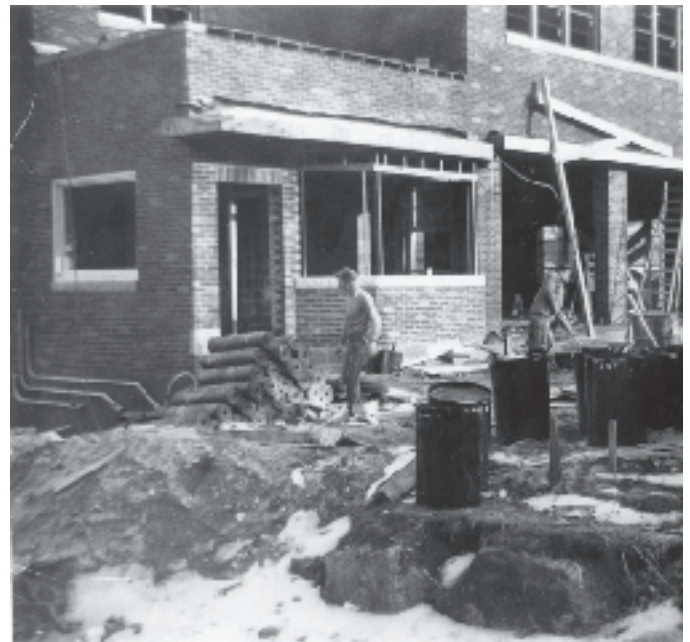
1952 Roofing materials for the Center Fire Station at 9 North Road. This building will be abandoned when the new Fire Headquarters opens at 50 Billerica Road in December 2014.
