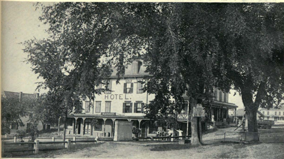
Central Square in the '90's, looking west and showing Wilson's Hotel Sweetser's Market, horse trough and the hay scales where the bubbler fountain now stands.
