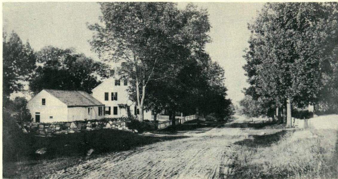
View down High Street about 50 years ago, showing the Solomon Parkhurst House.
