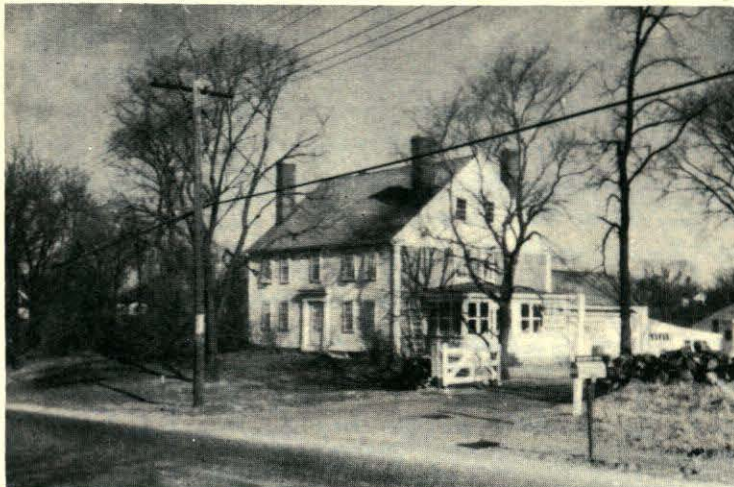
"Trooper Jock" Parker House at 134 Boston Road, Center.
