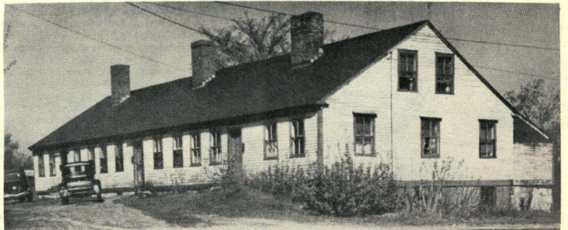
This is one of the houses of the Chelmsford Glass Works, a company established in 1802. There was at least one string of three units, a story and a half in height, each dwelling having a central chimney and two windows on either side of the door. It is highly likely that the housing was built shortly after the factory was started, for it was located in a very sparsely inhabited district. If that was the case, this would be the earliest American industrial housing development.
