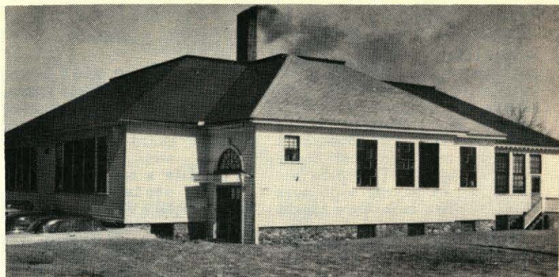
East School, East Chelmsford - now closed.
