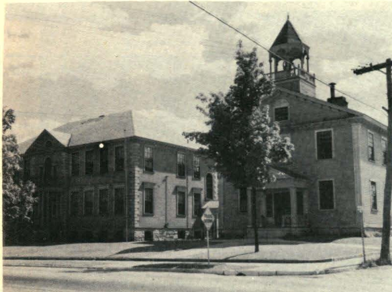
Princeton Street School which has been razed and a new fire house for North Chelmsford will be located on part of this land. The building on the right was constructed about the time of the Civil War while the building on the left was constructed about 60 years ago.
