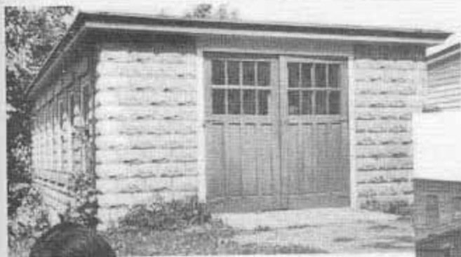
1920 Started business in this building Newfield St. No. Chelmsford
