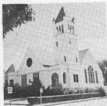
CONGREGATIONAL CHURCH North Chelmsford
