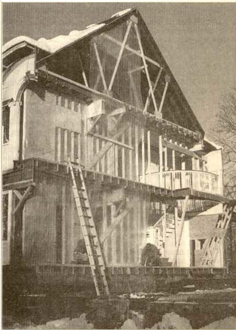
The Children's House was cut in half and wrapped in plastic recently. The actual move of the building should happen soon.
