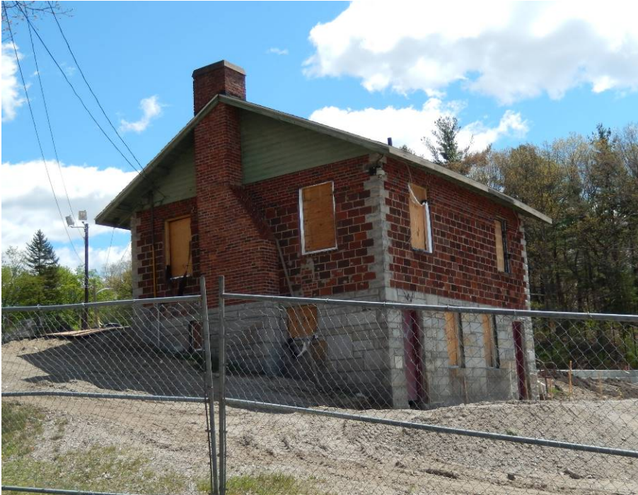
Rear of field house, facing southeast. May 2016.
