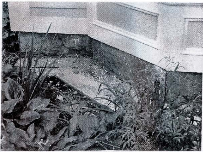
Typical granite block foundation under bay window
