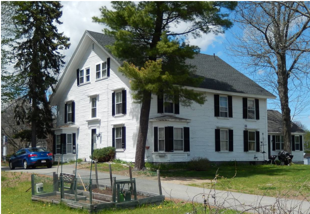
Rear and side walls, facing north. May 2016.
