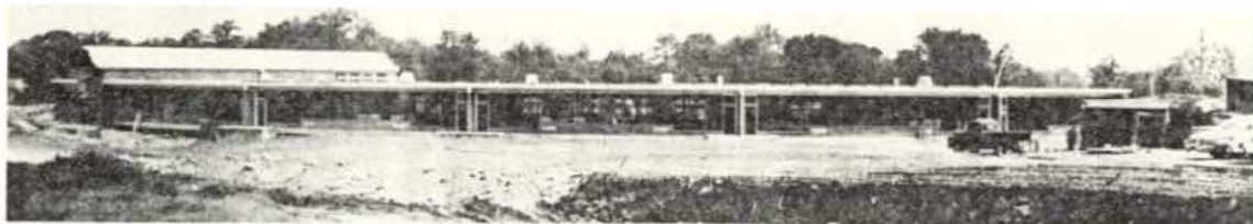
NEW CENTER SCHOOL TAKING SHAPE - Picture taken from Billerica St. shows the new Center school which is being built by the Vara Construction Co. It is expected that the building will be completed some time in December with hopes that it may be sooner.
