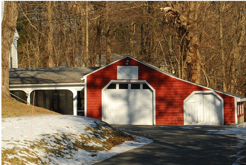
Garage. View looking east.
