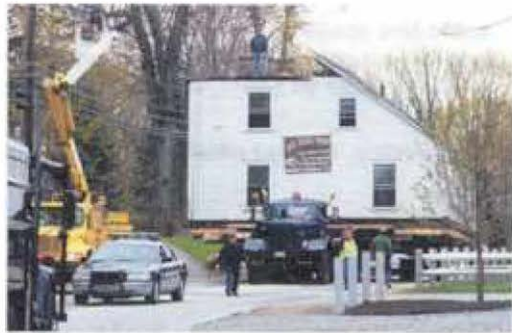
MOBILE HOME: Workers move utility lines as the Hill Jock House crawls down Boston Road in Chelmsford yesterday to its new site on Garrison Road. SUN / BILL BRIDGEFORD
