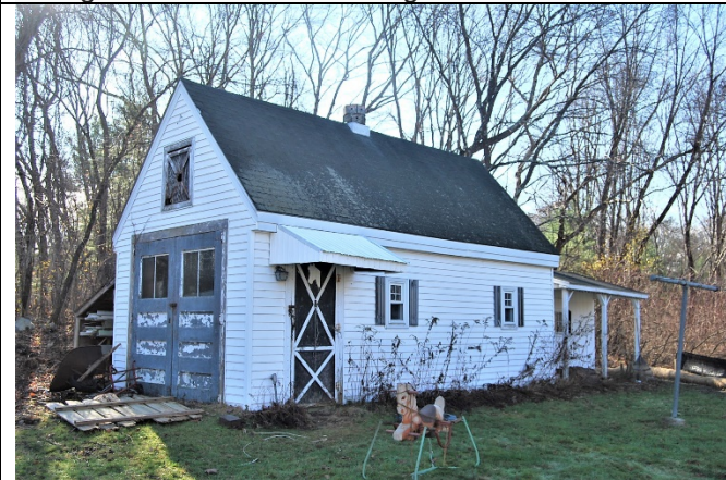
Shed. View looking south.
