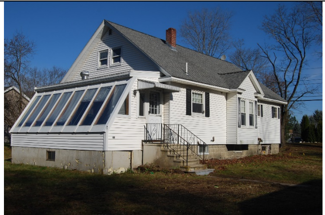
Southwest and southeast elevations. View looking north.
