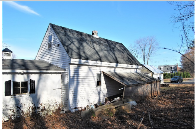
Shed. View looking north.
