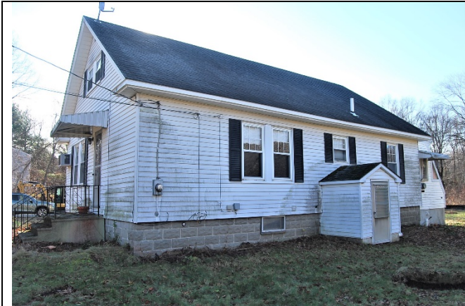
Northeast and northwest elevations. View looking south.
