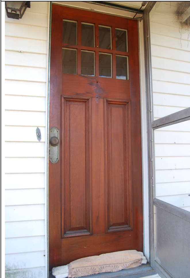
Entry door. Façade (northeast elevation).
