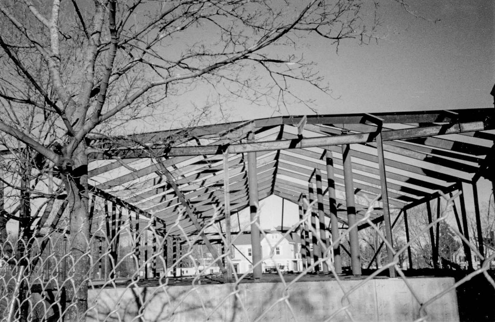
25 Boston Road - Chelmsford Public Library addition construction 12/21/1998
