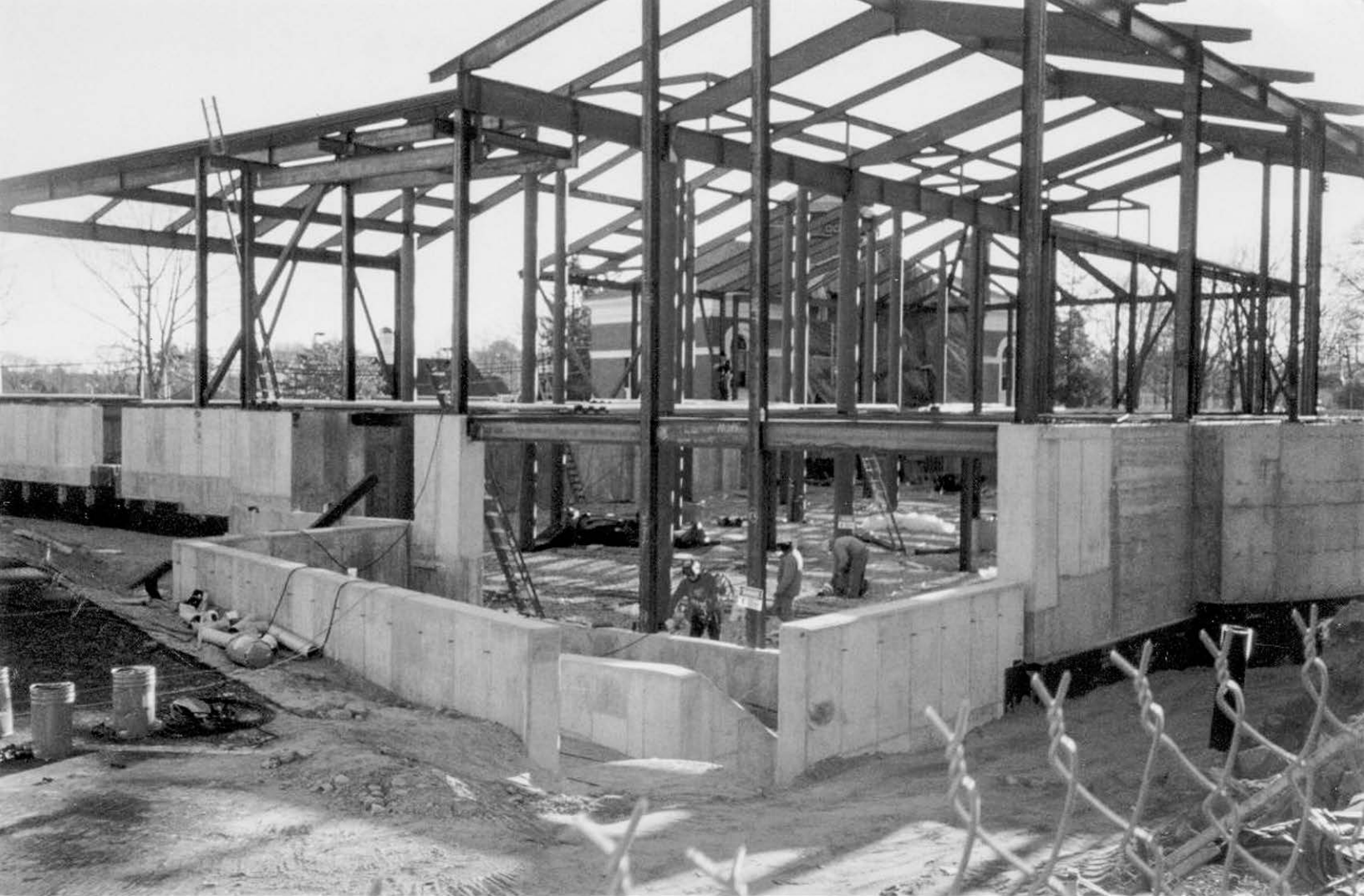
25 Boston Road - Chelmsford Public Library addition construction 12/21/1998
