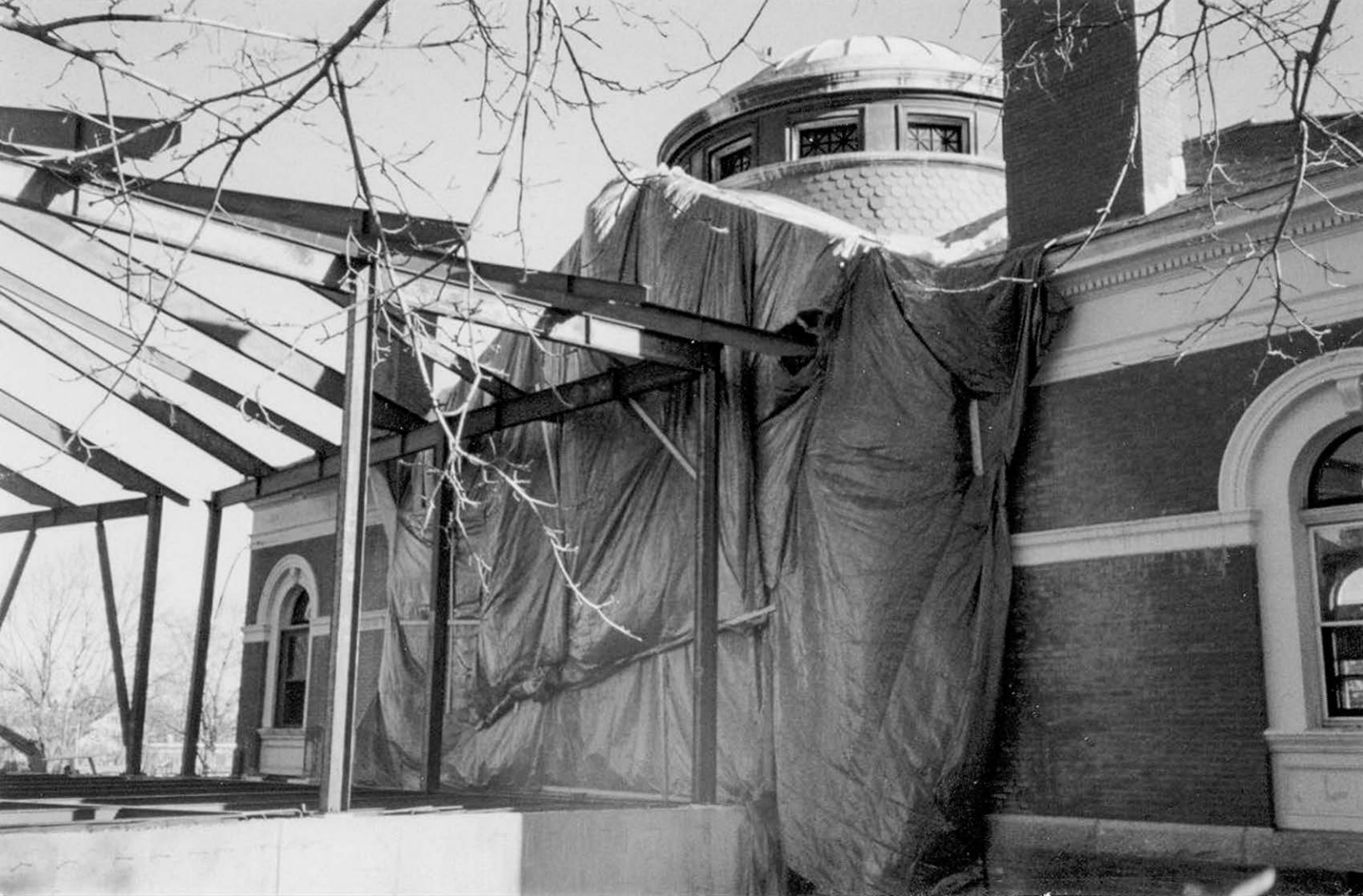
25 Boston Road - Chelmsford Public Library addition construction 12/21/1998
