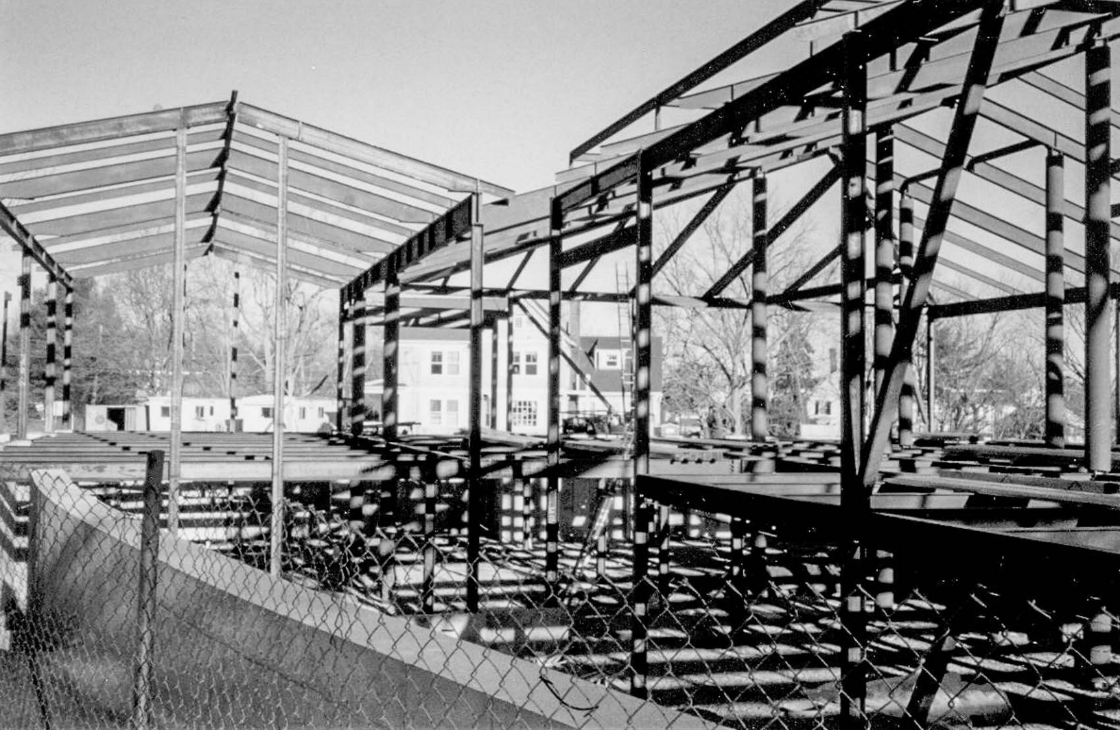
25 Boston Road - Chelmsford Public Library addition construction 12/21/1998
