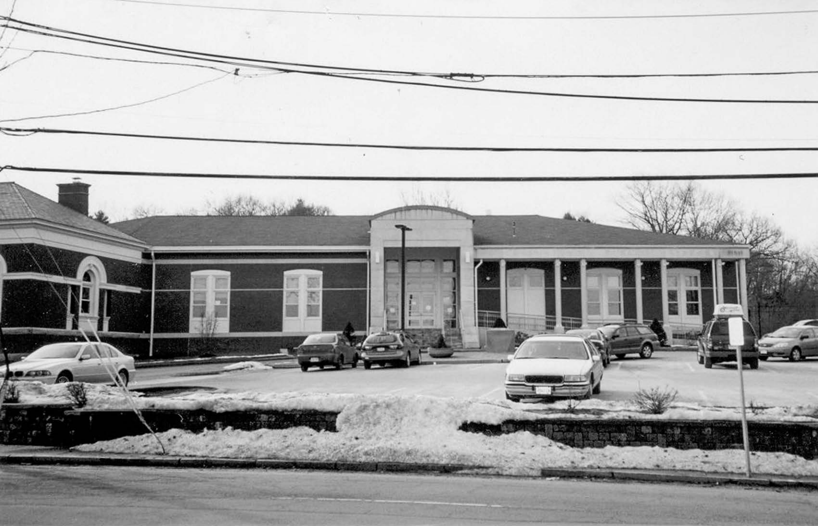
25 Boston Road - Chelmsford Public Library addition to Adams Library
