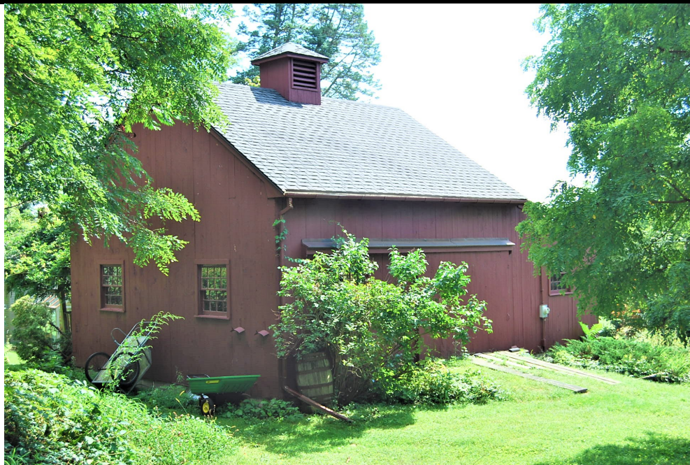
Barn/Garage, north and west elevations. View looking southeast.
