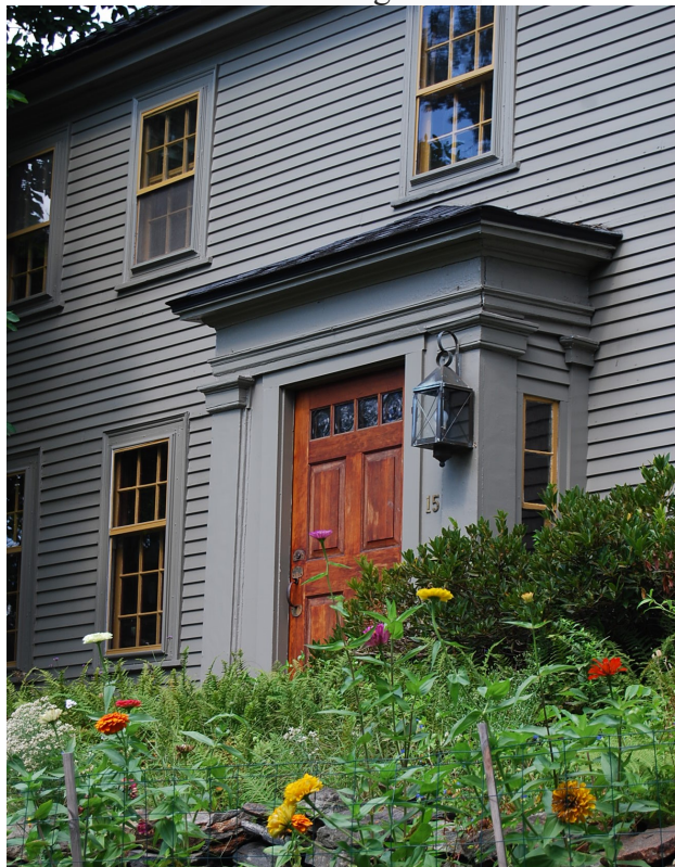
Entrance detail. View looking northwest.
