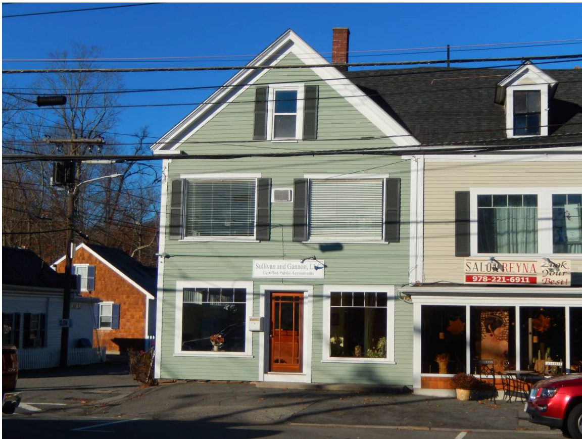
22 Central Square, facing west. November 2015.
