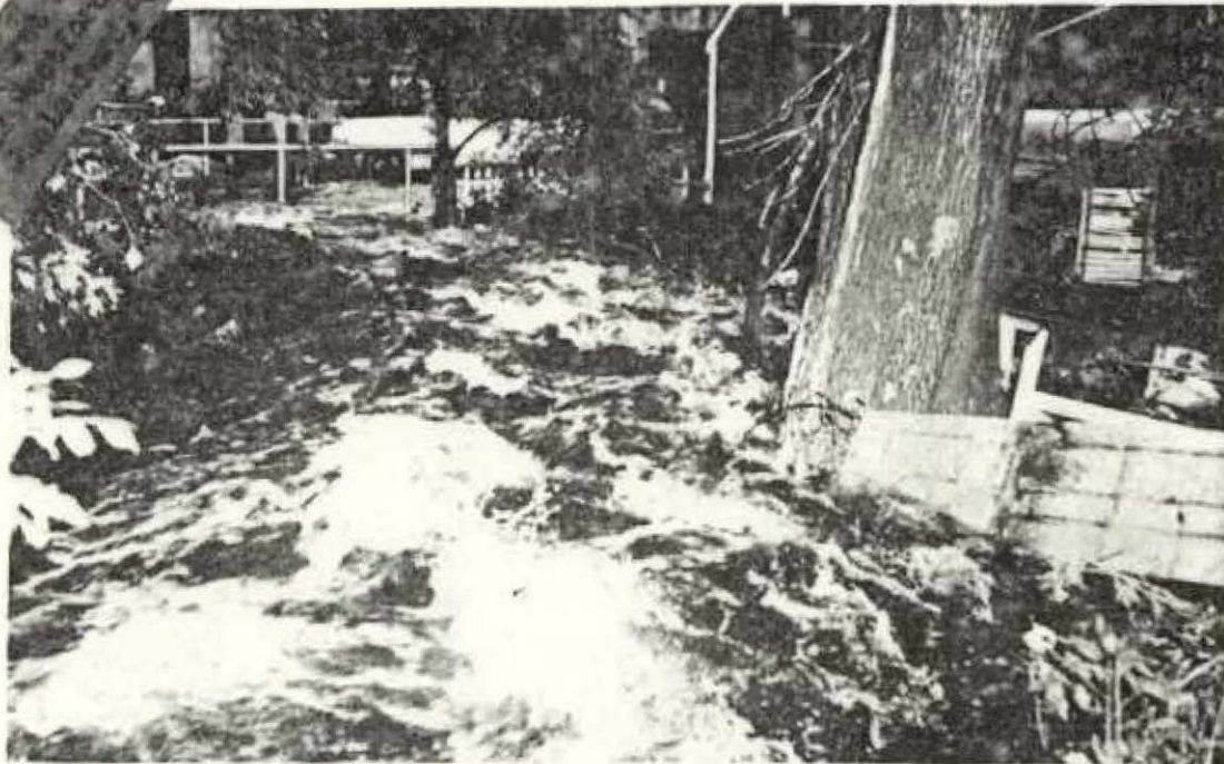
A VIEW OF BEAVER BROOK in the rear of the Old Mill House in Central Square on Saturday evening after Hurricane Edna had struck. Note the rail of the bridge which was installed last year.
