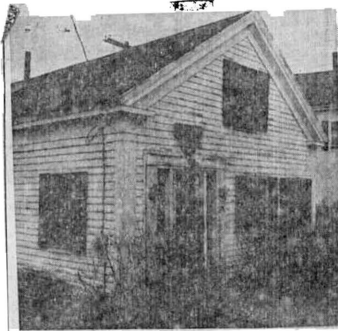
The centrally located historic property known as the Mill House is being considered for purchase by the town of Chelmsford.
