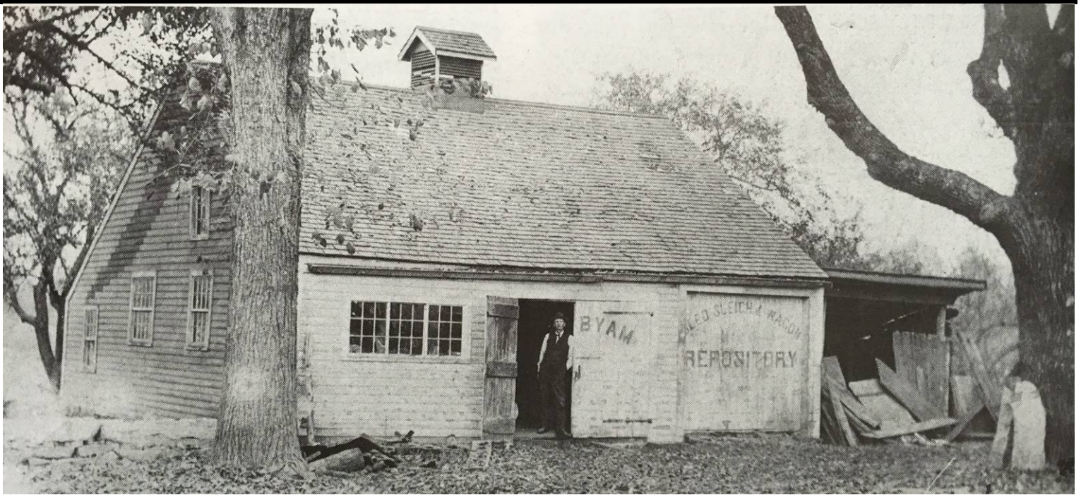
1908 photograph of the blacksmith shop in its original location on Maple Road. (Chelmsford Historical Commission/ Linda Prescott.)
