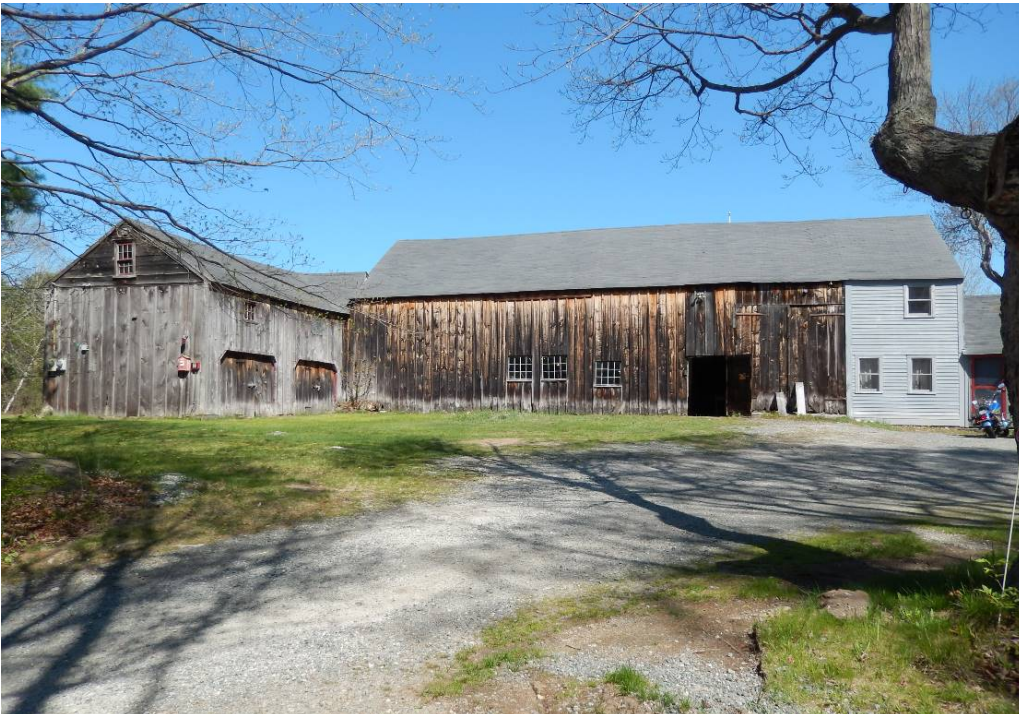
Garrison House Barn, CLM.340, facing north. May 2016.
