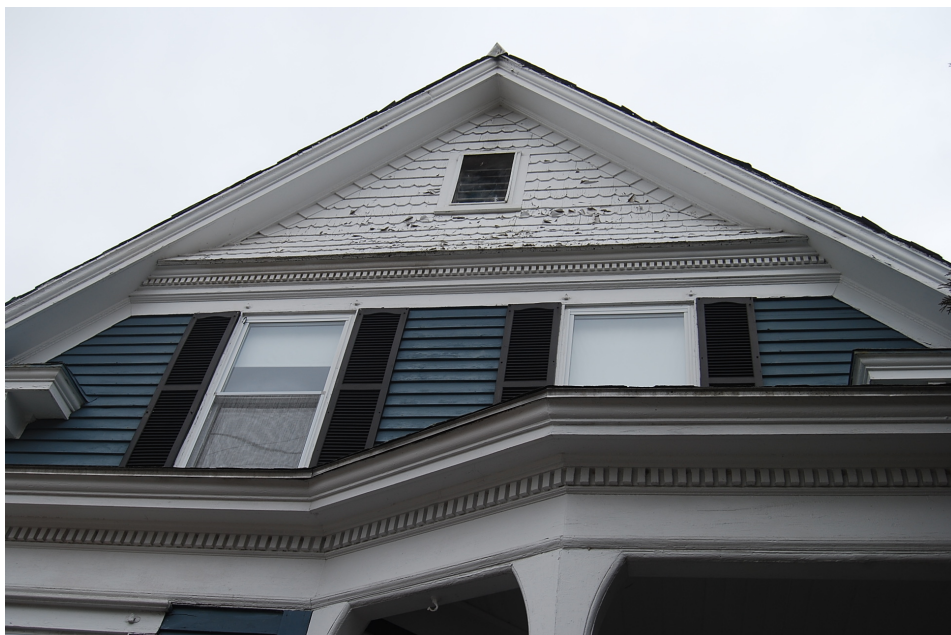
Photo 4. Detail. East façade.
