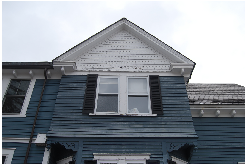
Photo 8. Detail. South elevation projection.
