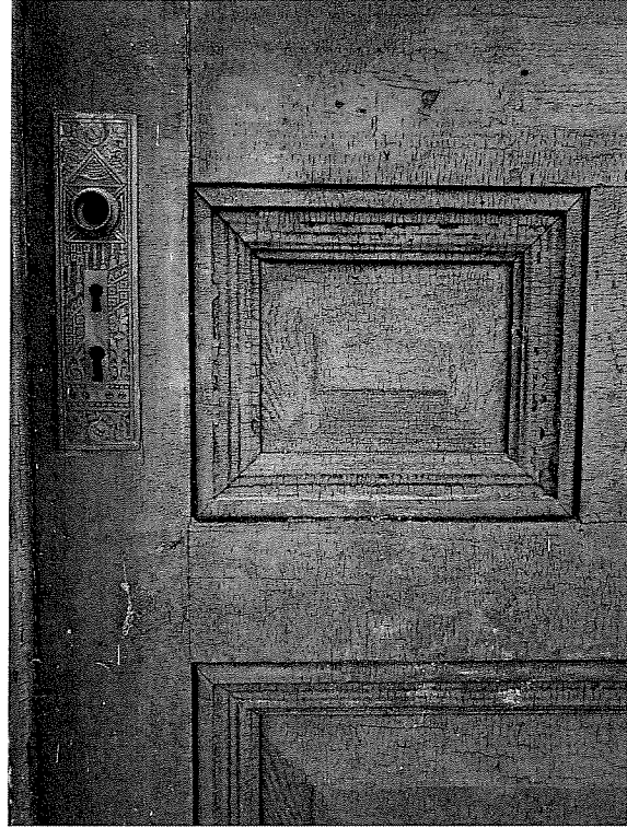
Detail. Main door, north elevation.
