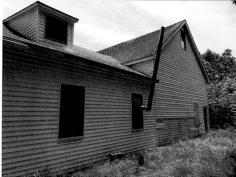
View looking southeast. West elevation. Garage at left. Barn at right.
