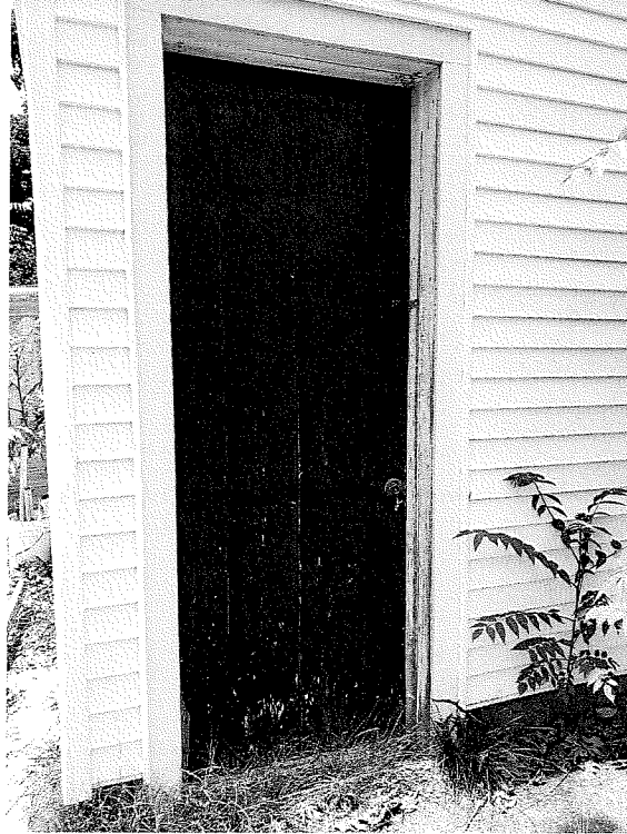
View looking west. Barn, east elevation.
