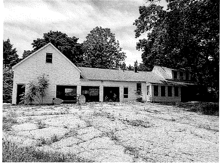
View looking west. House is at far right.
