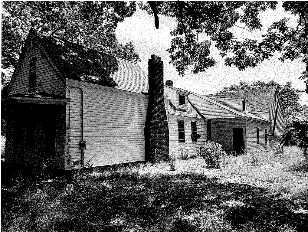
View looking southeast. From left to right: House, ell, garage, barn.
