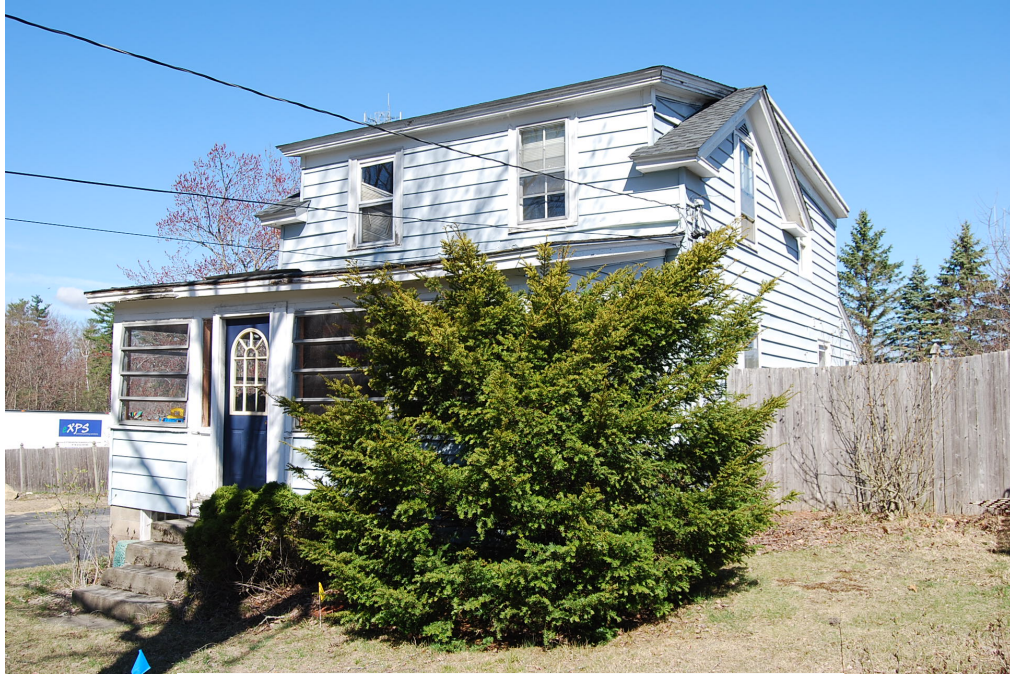
South and east elevations. View looking northwest.
