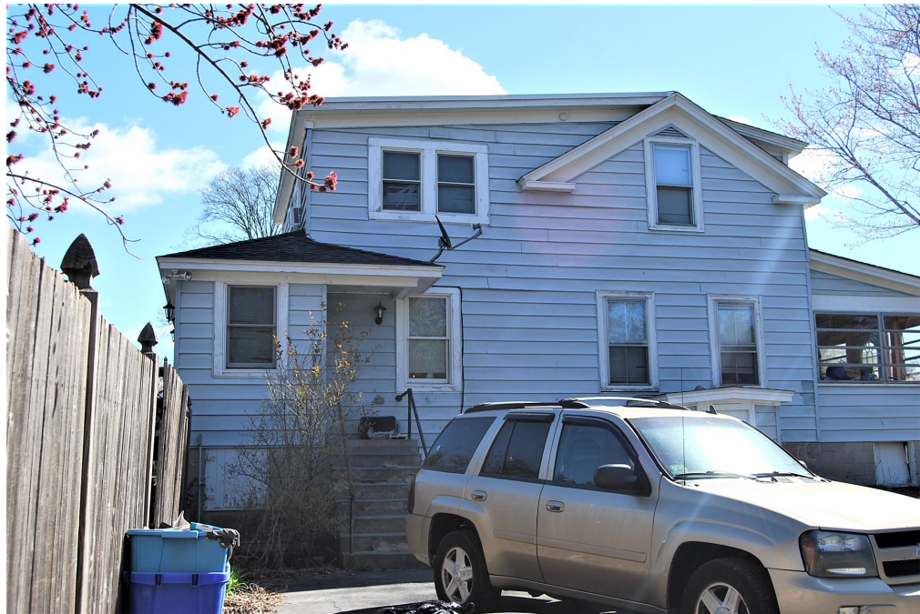
West elevation. View looking east.
