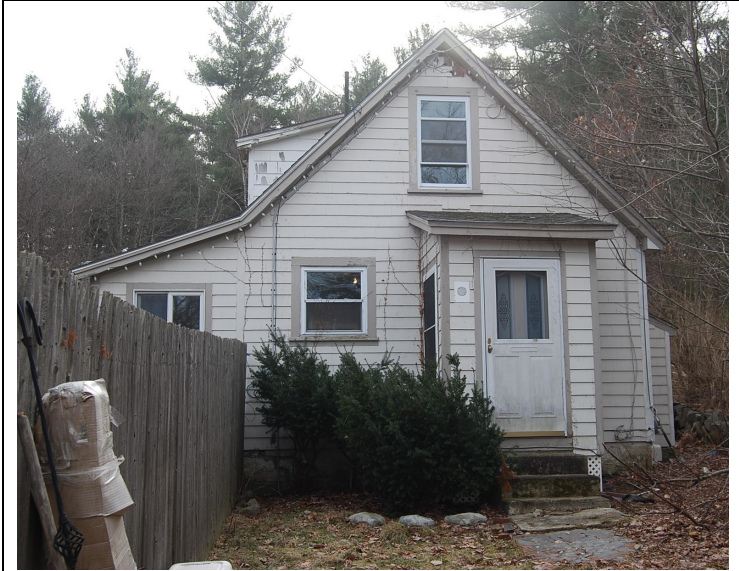
North Façade. View looking southeast.
