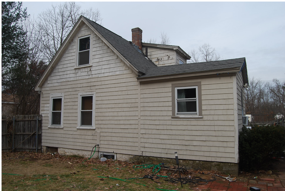
Rear, south elevation. View looking northwest.
