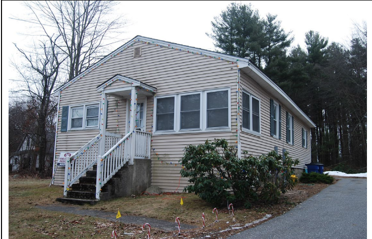
North façade. View looking southeast.
