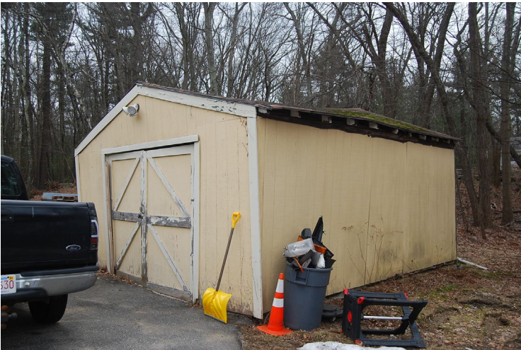
Garage. East and north elevations.
