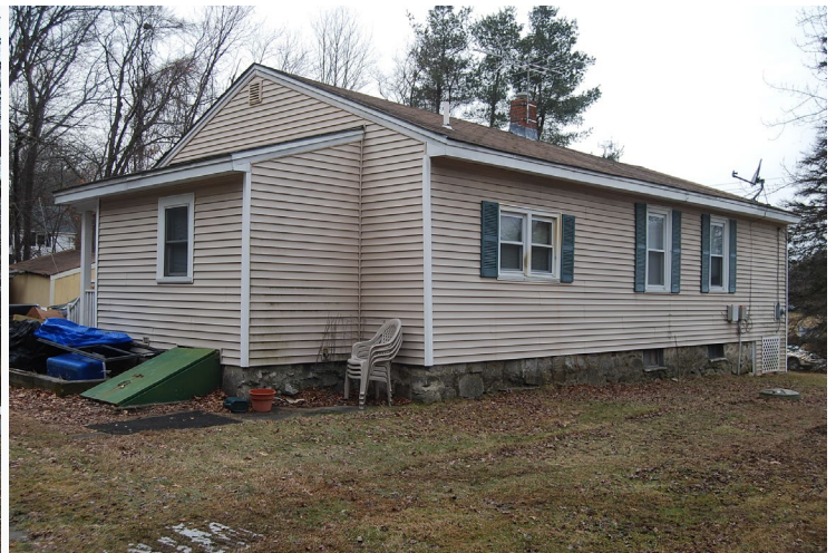
South and East elevations. View looking northwest.
