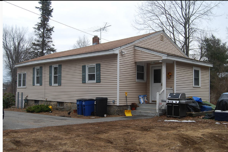
West and South elevations. View looking northeast.
