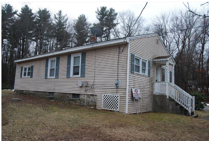
East and North elevations. View looking southwest.
