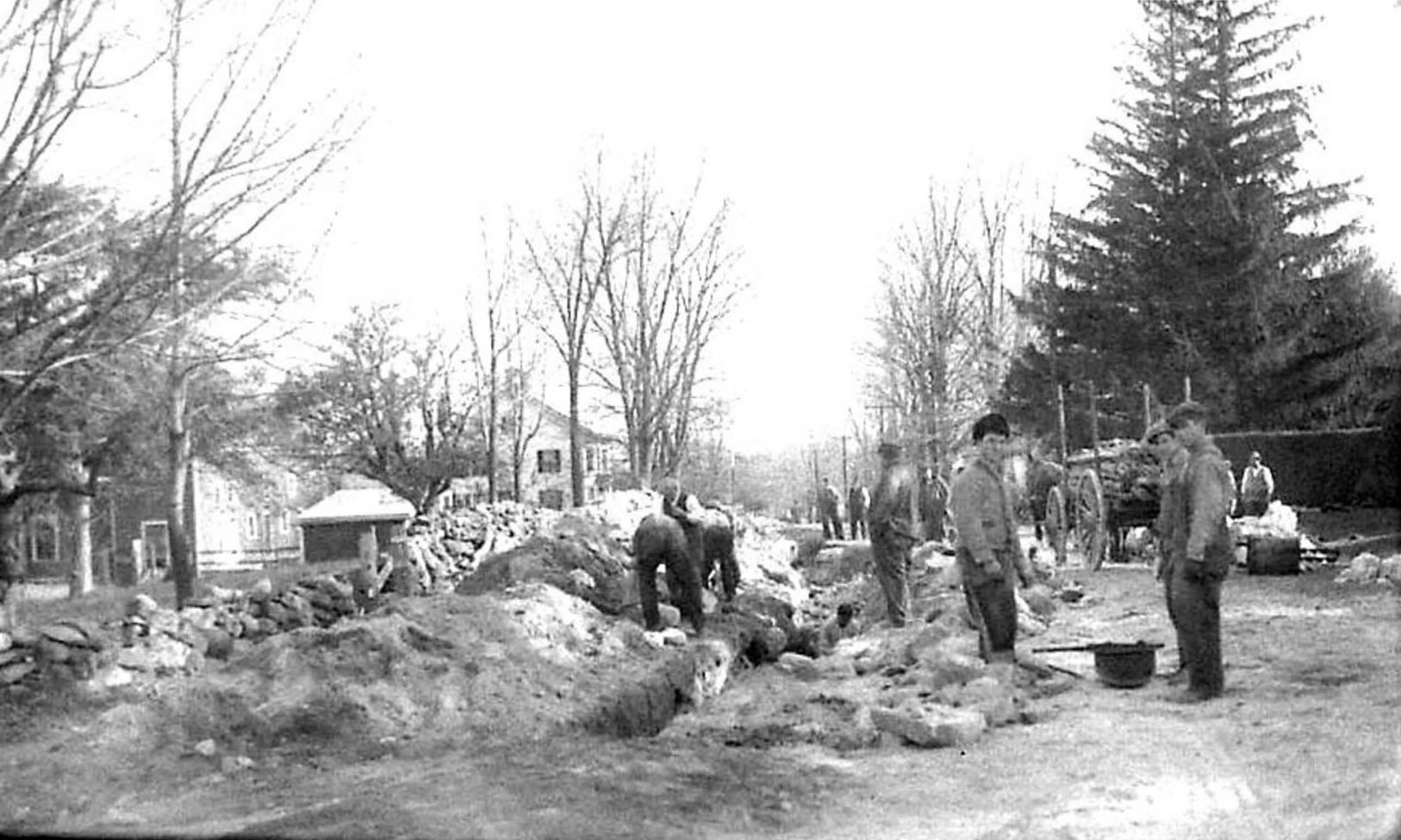
Installing water pipe in front of 78 High Street
