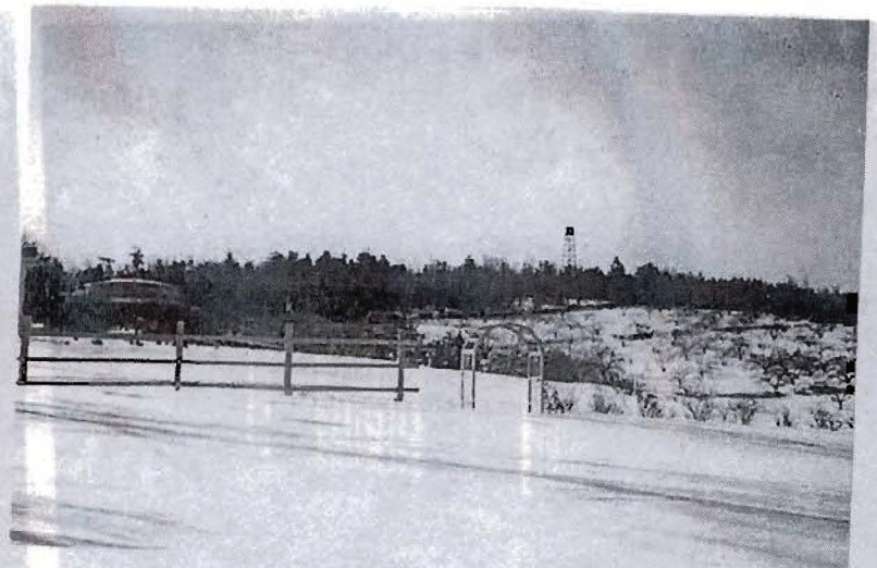
1942 From driveway Toward Robin Hill Tower
