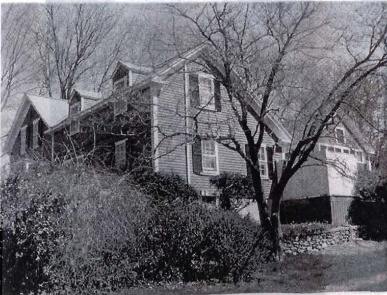
Main house Addition ↑
