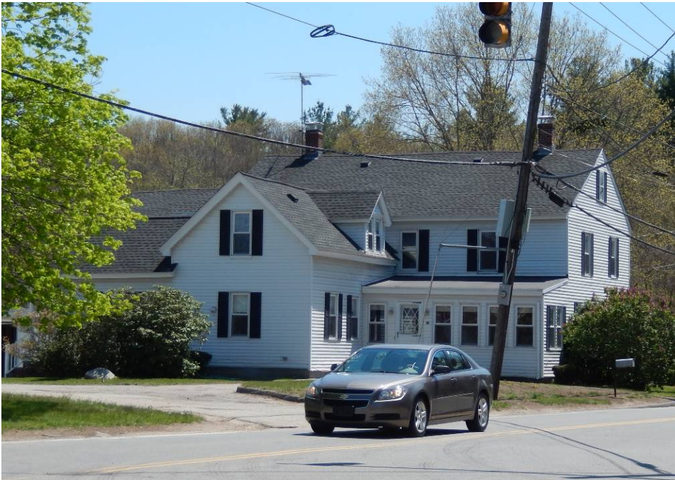
Rear of 50 Hunt Road, facing south. May 2016.
