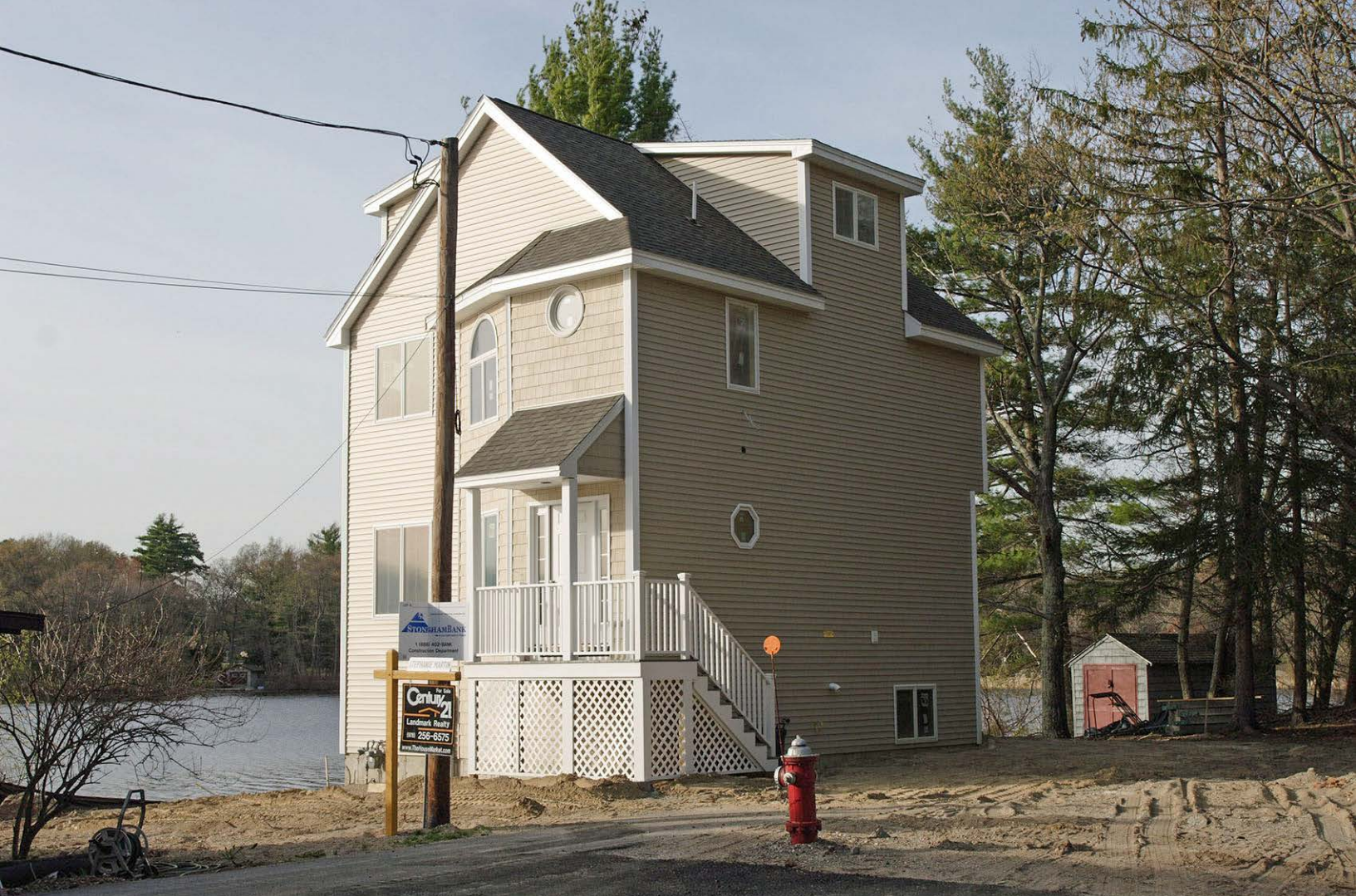
1 Lakeside Avenue after demolition and rebuild
