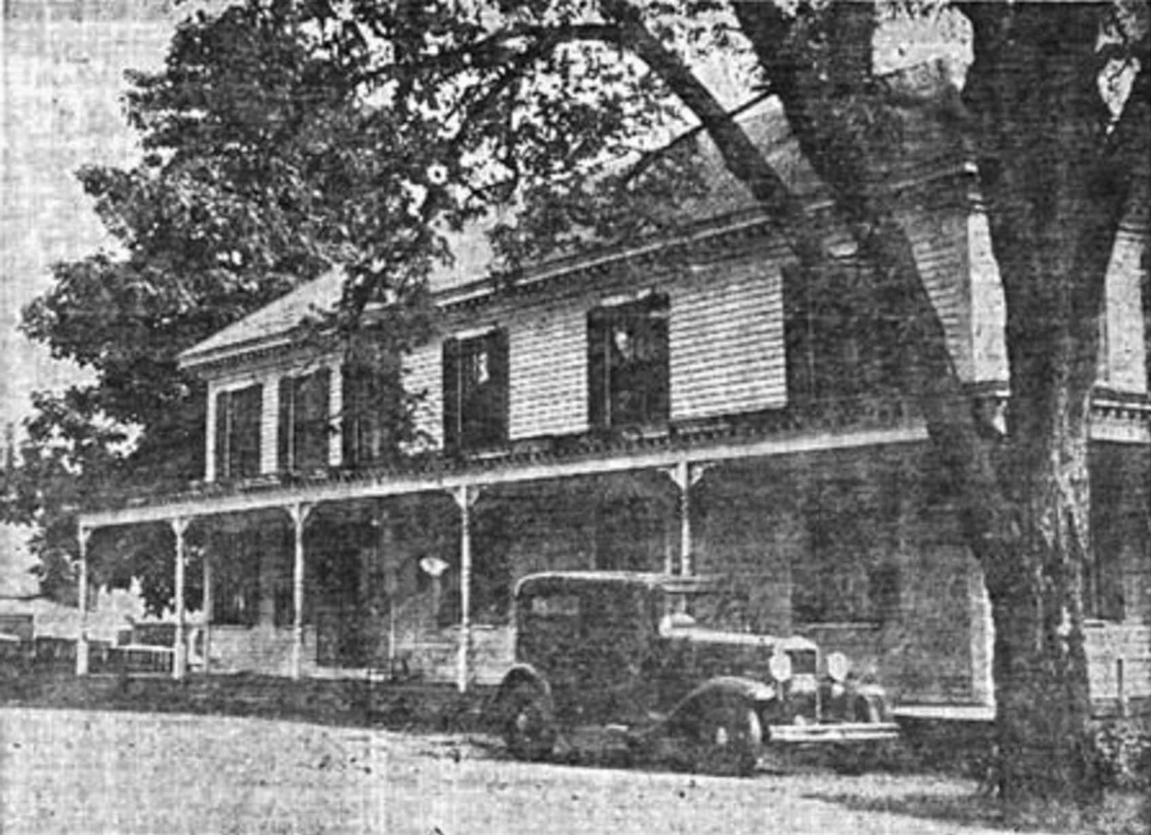
1677 Railroad House - demolished in 1937
