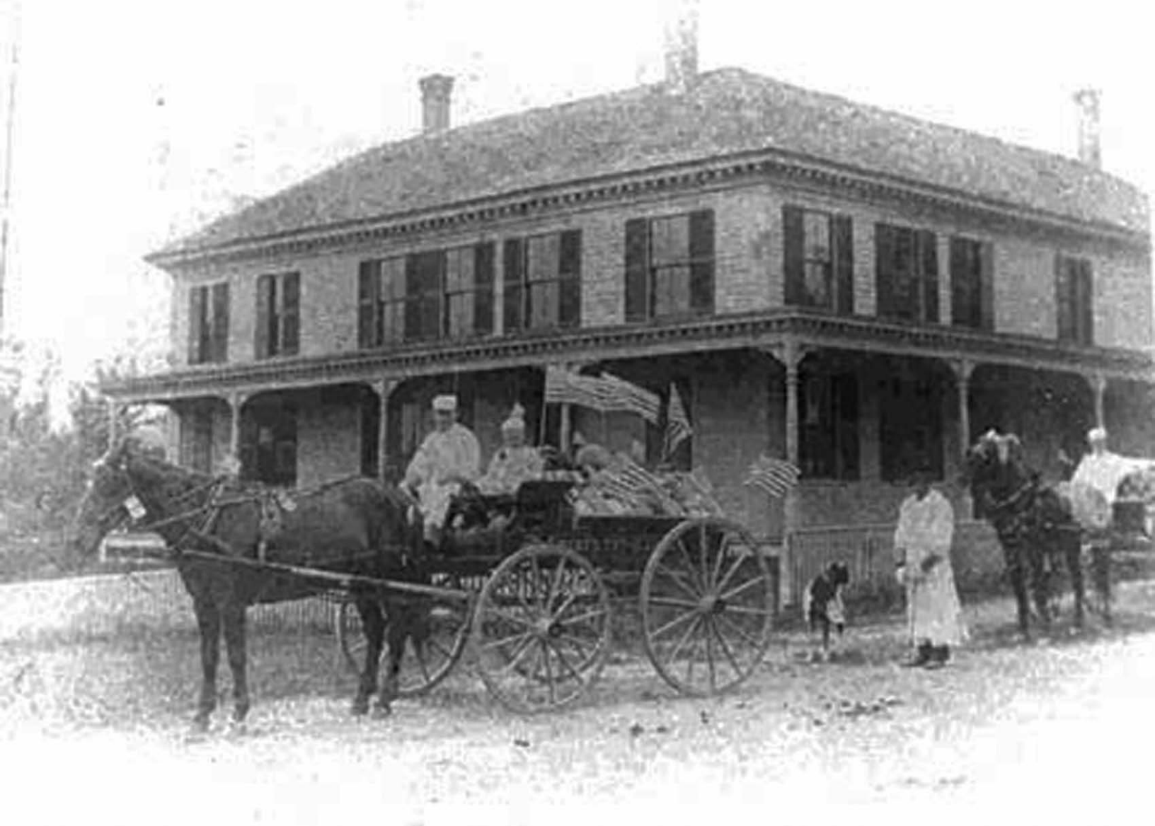
1677 Railroad House - Demolished by Chelmsford Ginger Ale in 1937 to make room for expansion
