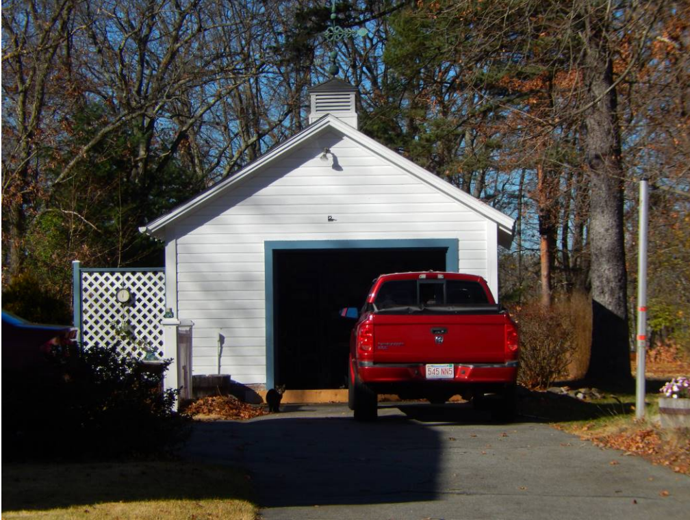
Garage, facing north. November 2015.
