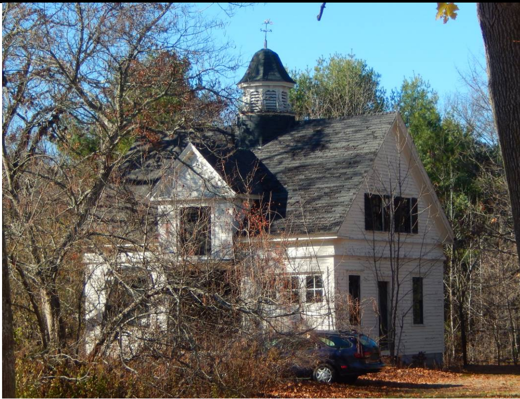
Carriage house, facing northwest. November 2015.
