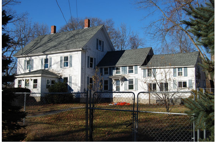
View looking northwest from Manning Road.
