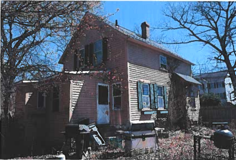
North elevation and ell at left; west elevation at right. View looking southeast.
