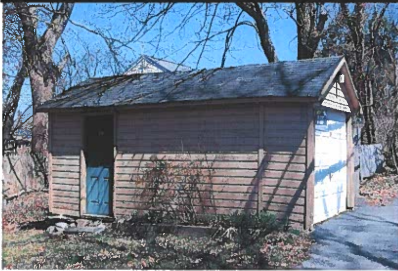
Garage west elevation and façade (south) elevation. View looking east.
