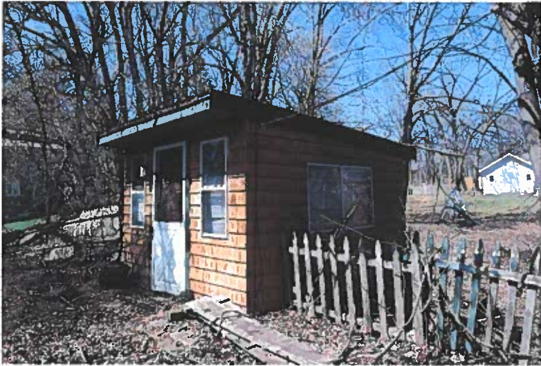
Shed. View looking northwest.
