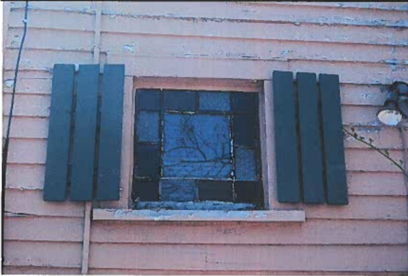
Multi-color, pressed glass window on east elevation.
