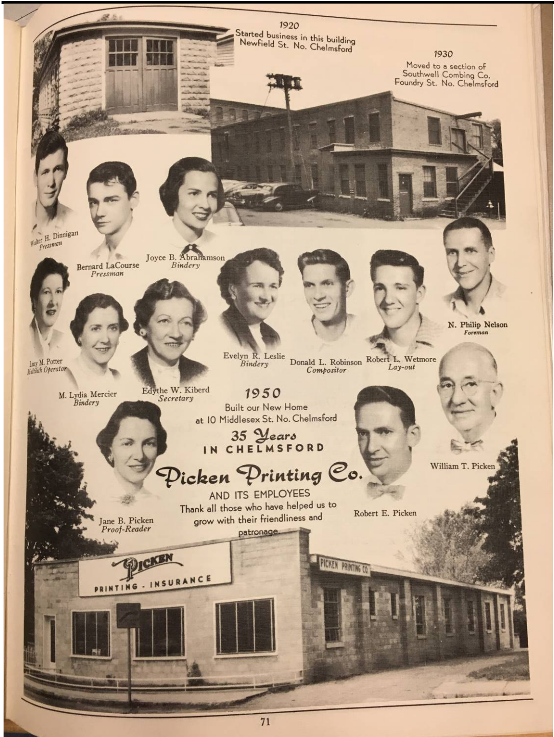
From the Official Tercentenary Souvenir Program 1655-1955, showing previous locations of the company and the building at 10 Middlesex Street, as constructed in 1950. Available at the Chelmsford Public Library.
