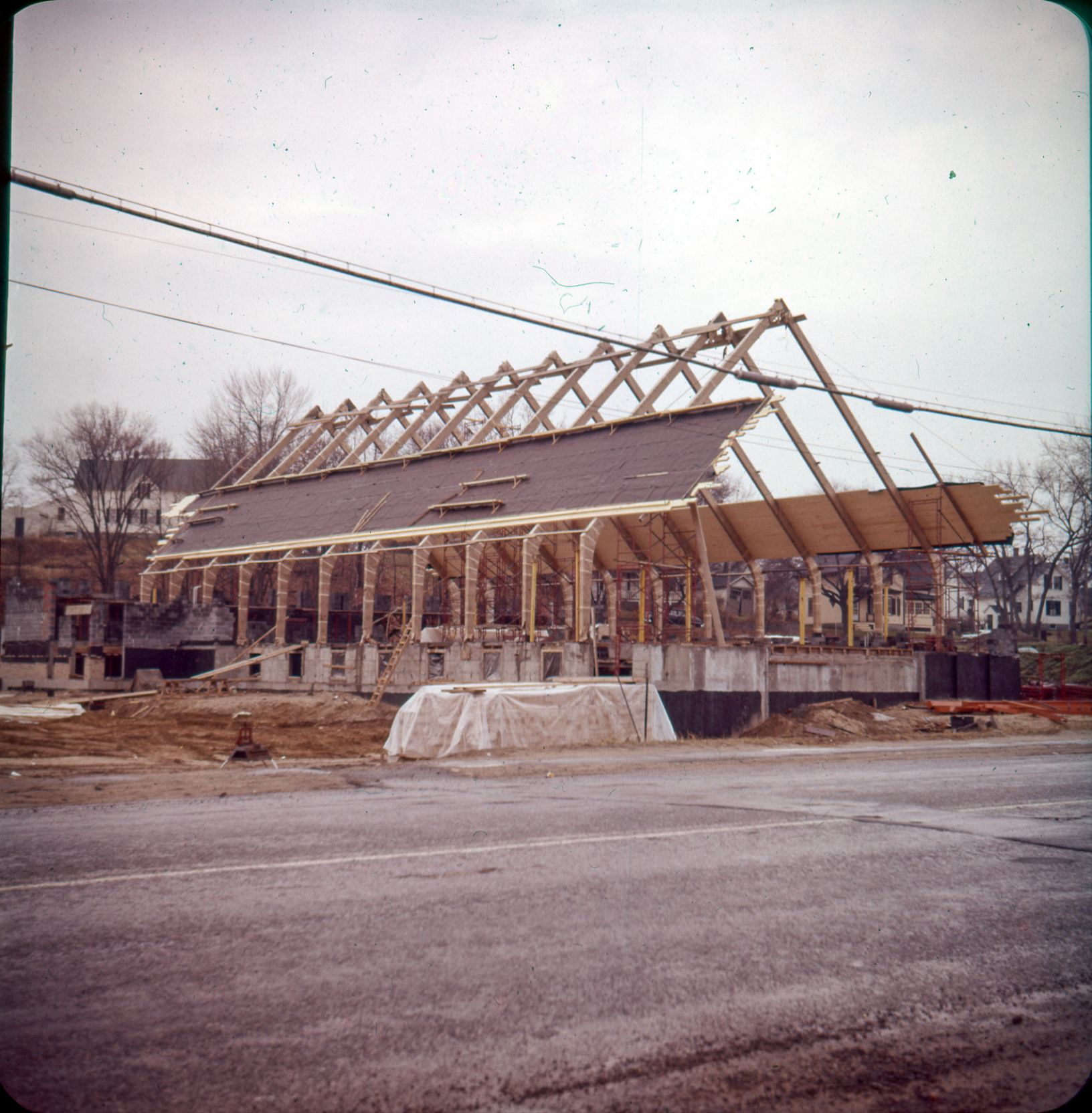
This series of construction photos courtesy of Liliana Lucas, Saint John's church, North Chelmsford
