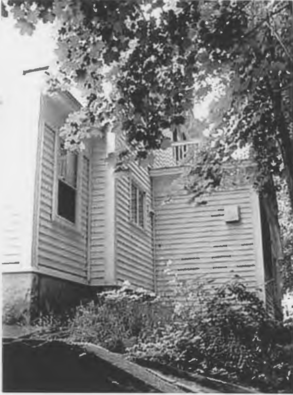
North wall looking east Left side of house
