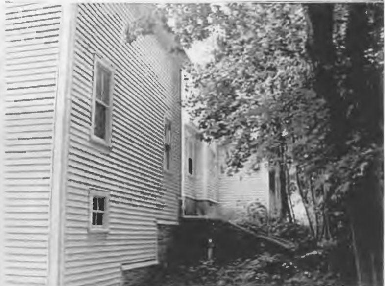
North wall of barn-connecting area-main house
