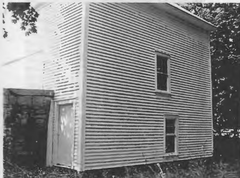
South side of barn rear of barn
