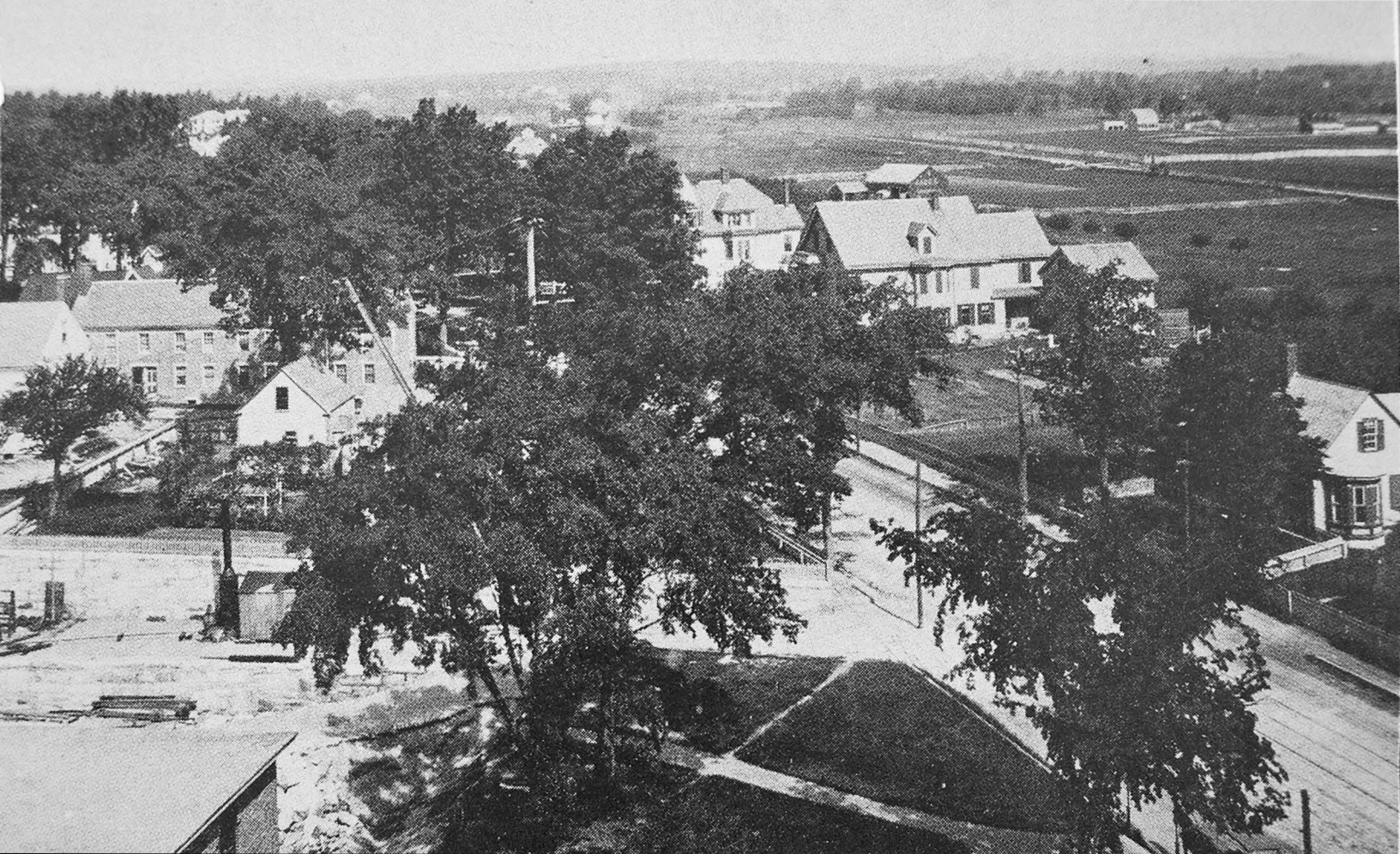
View from roof of Silesia Mill, 54 Middlesex Street of far right
