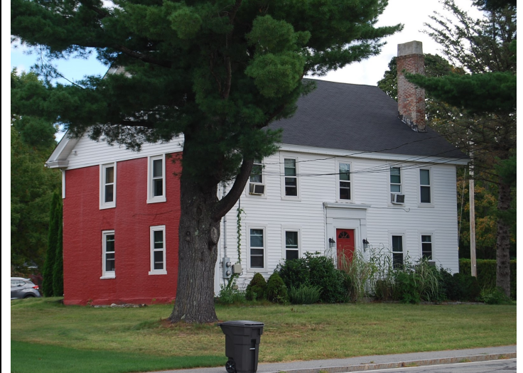
View looking northeast from Mill Road.
