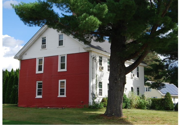
View looking northeast. West (side) brick elevation.
