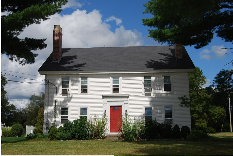
View looking north. Façade.
