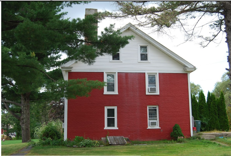
View looking west at east elevation.
