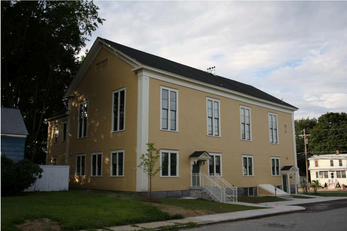
North Town hall before and after photos by Fred Merriam
