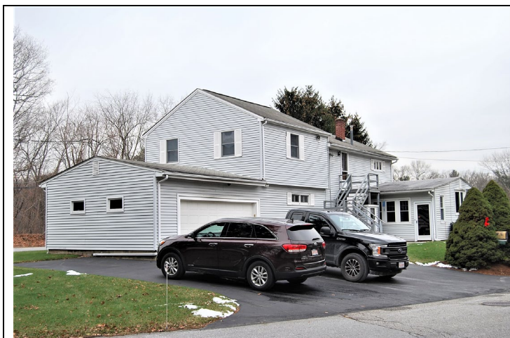
View looking northwest from Fairview Street.
