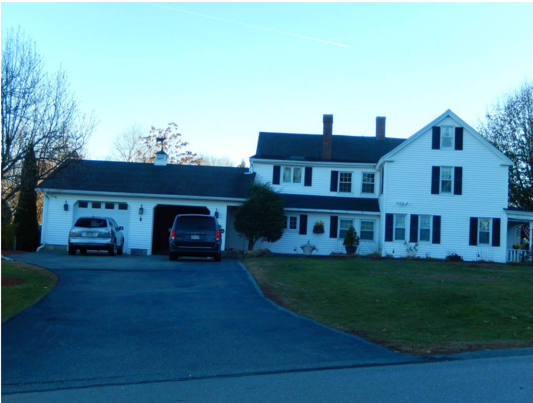
147 North Road, facing southeast, taken from Wiggin Street. November 2015.
