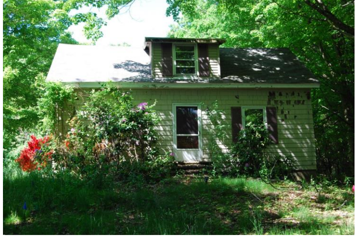
View looking southwest toward façade.
