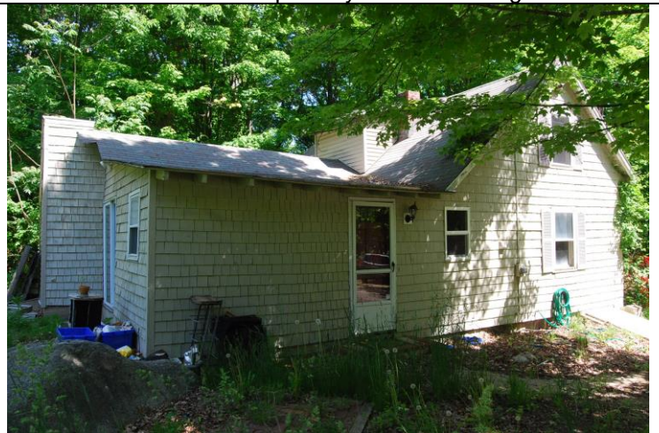
View looking north toward southeast elevation. Enclosed porch visible at left.
