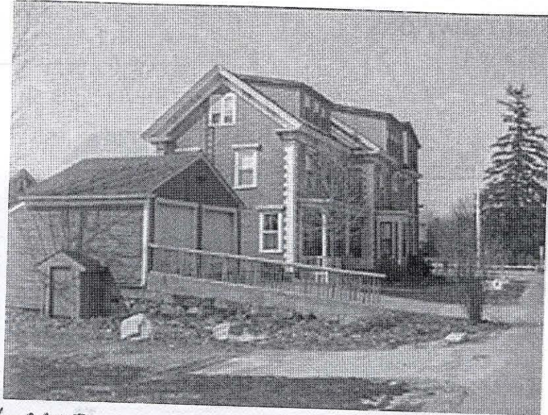
garage left + front of house
