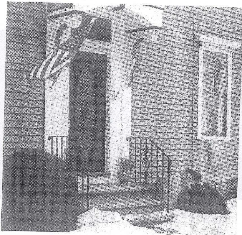
Front door + windows before changes 2001
