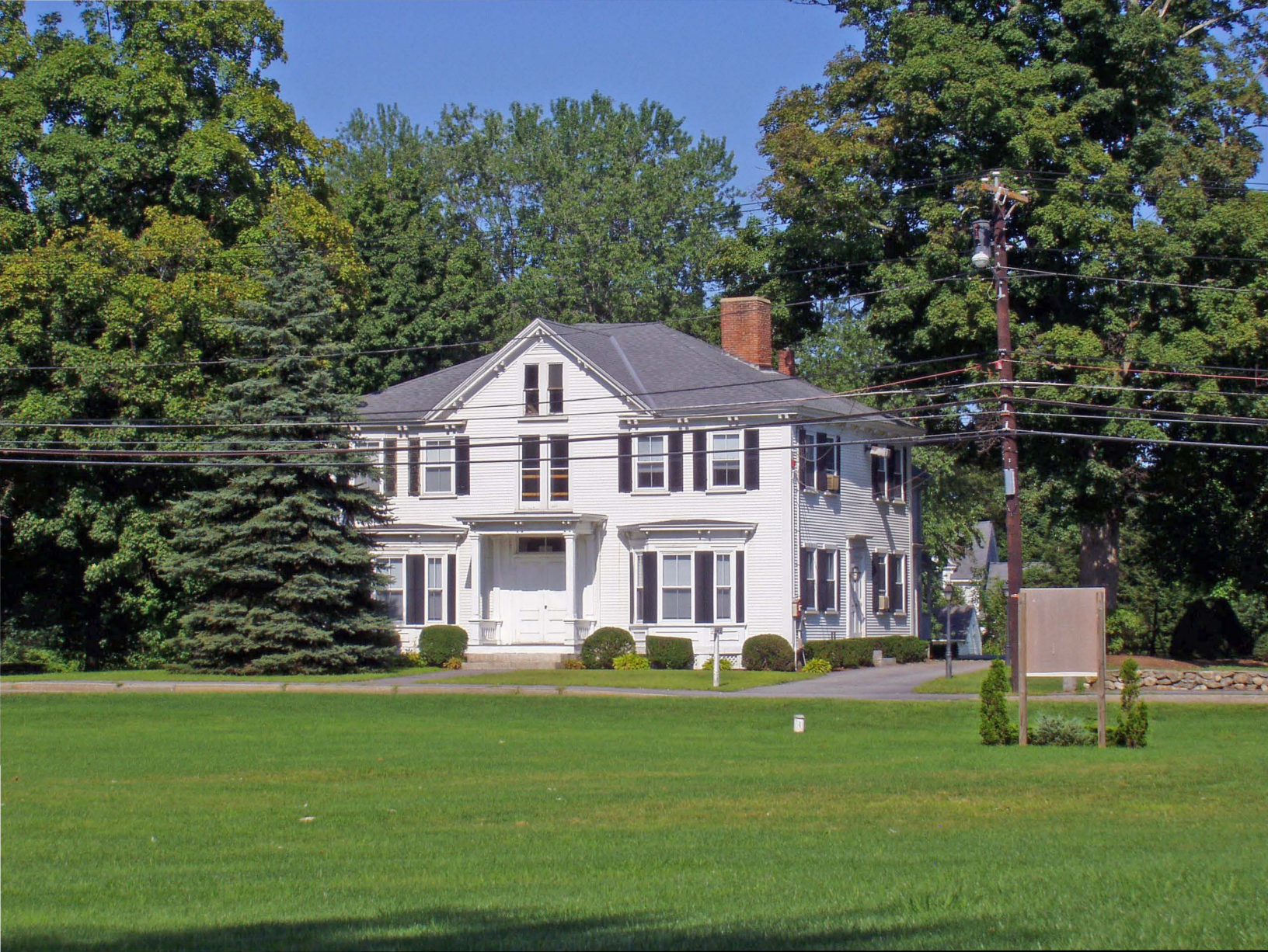
33 North Road - History lost across the street
