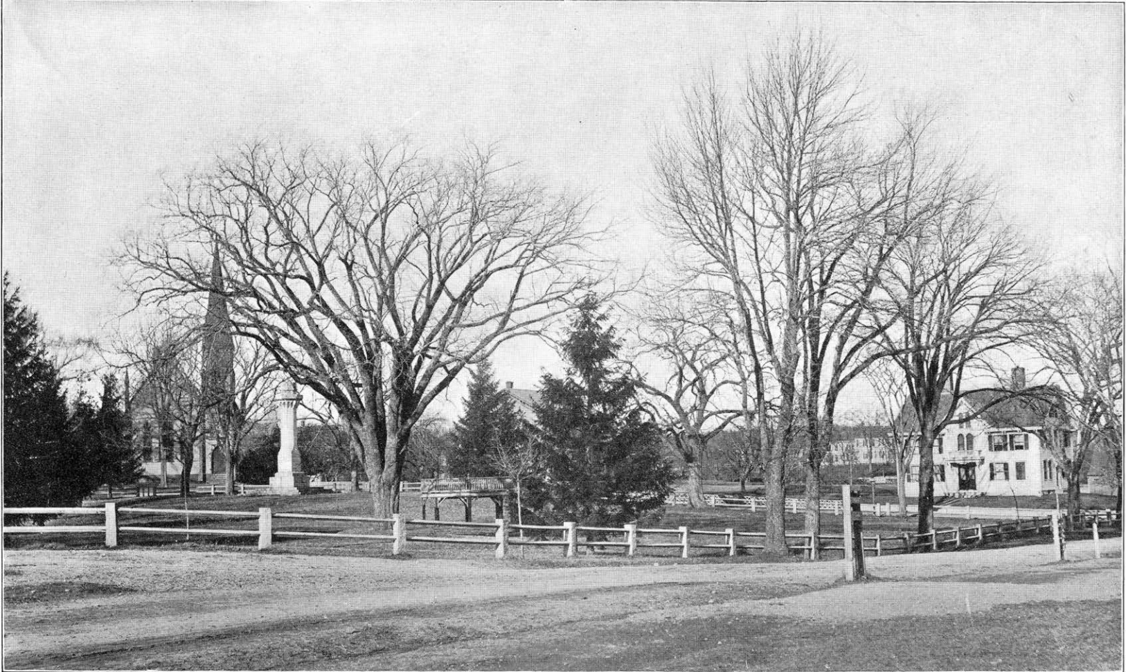
6 North Road on right
