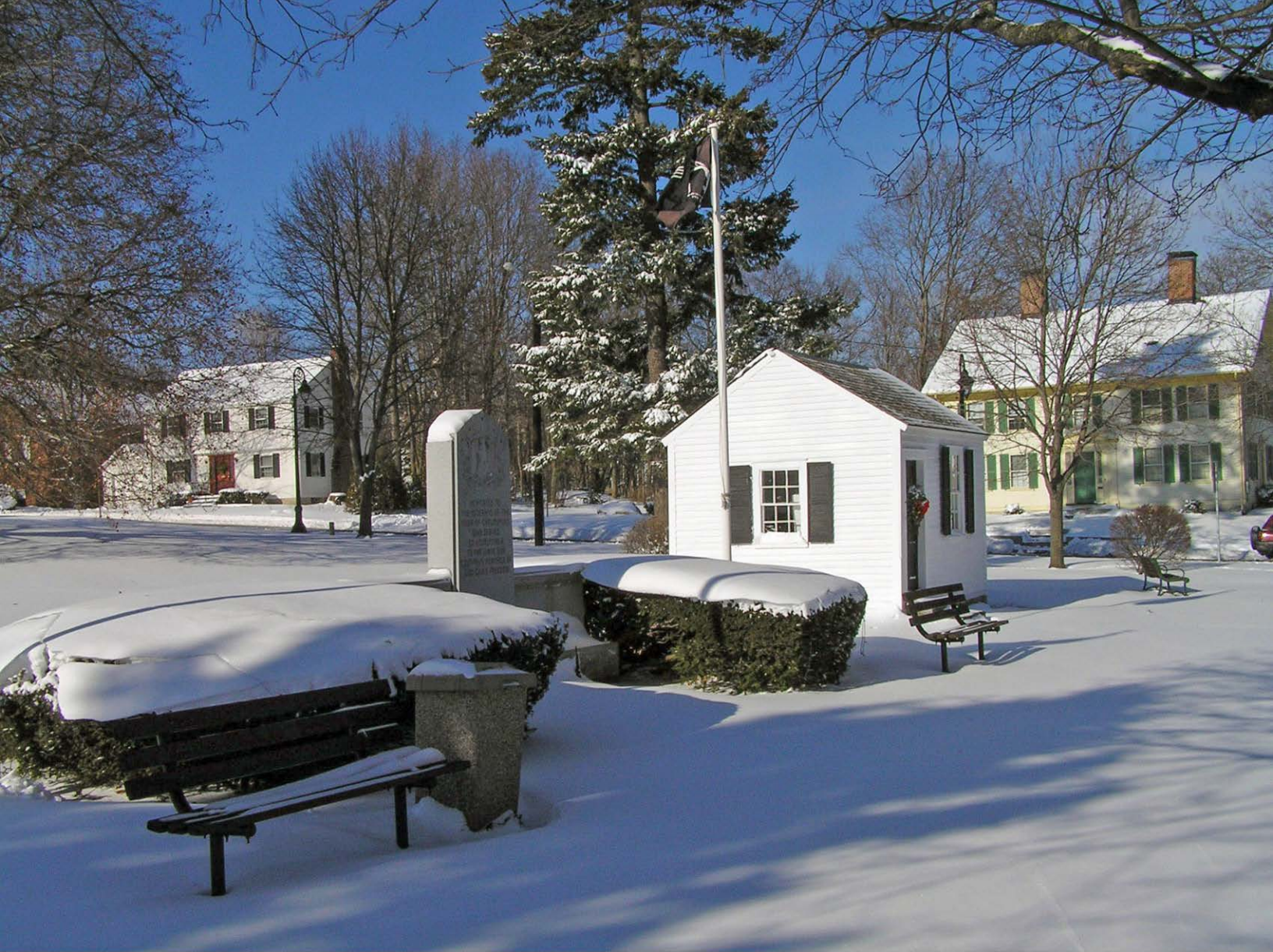
North Road - Middlesex Canal Toll House
