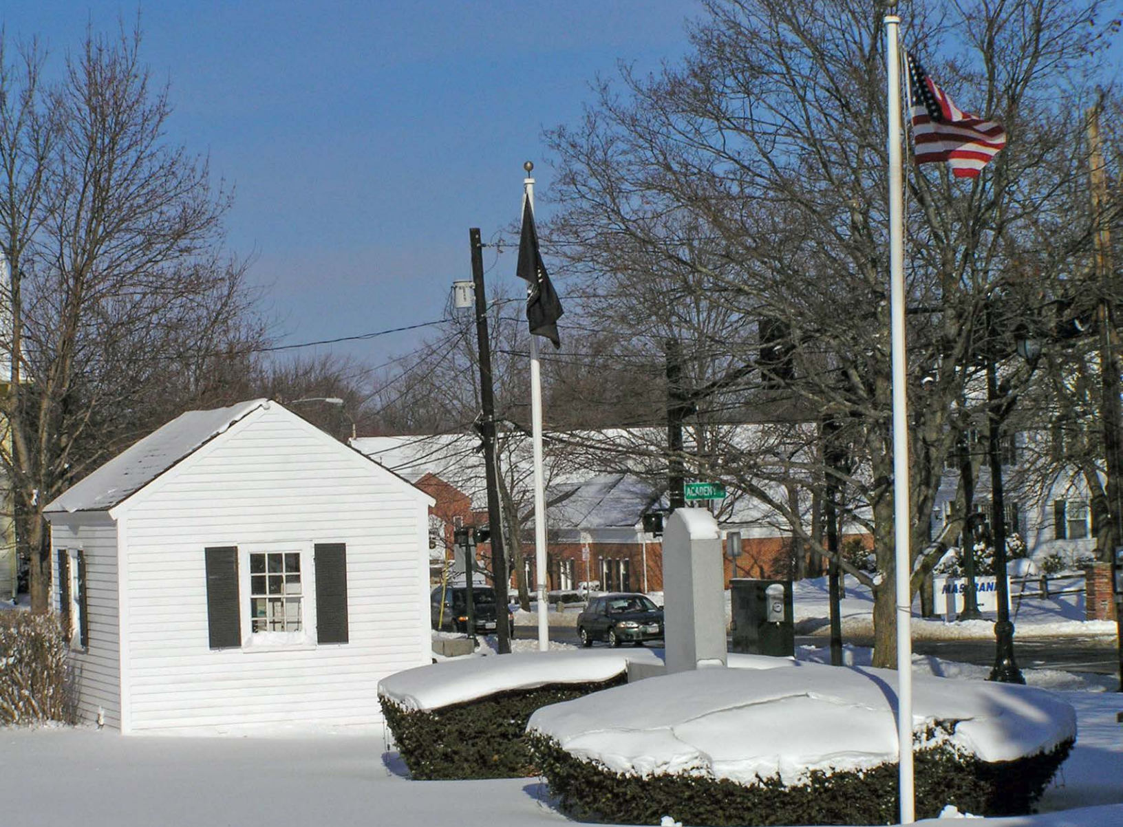
North Road, Middlesex Canal Toll House
