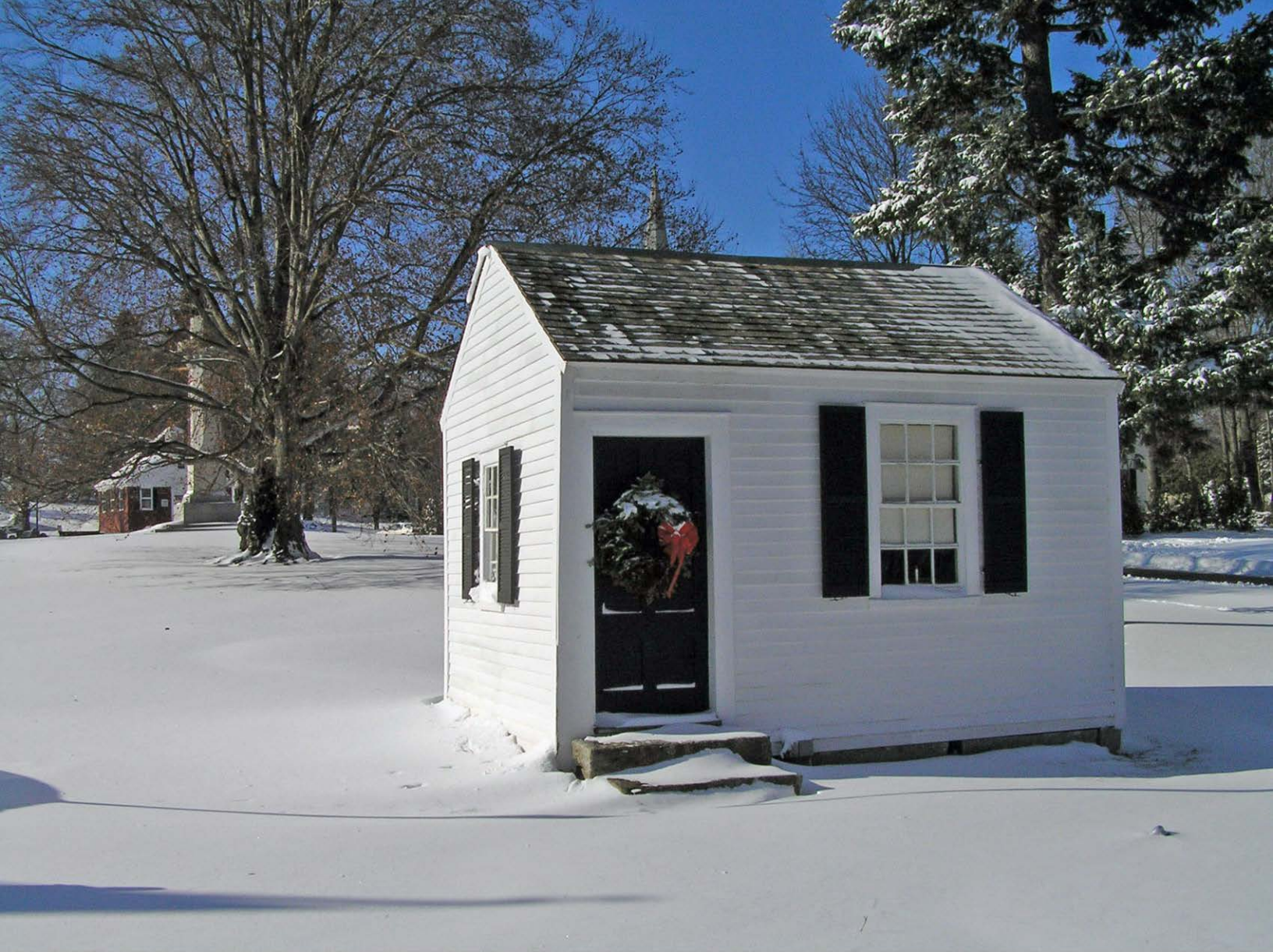
North Road - Middlesex Canal Toll House
