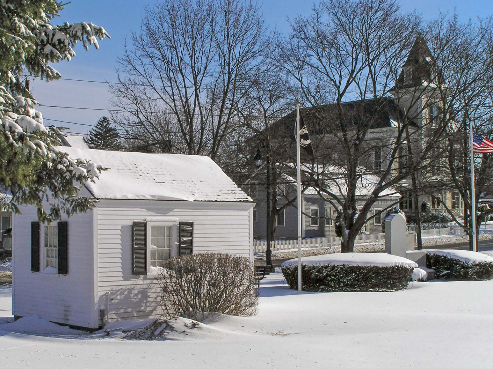
North Road - Middlesex Canal Toll House
