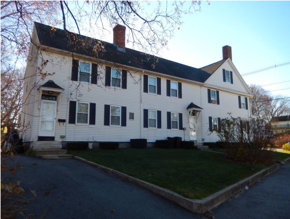
Rear ell of 22-28 Princeton Street, taken from Wright Street, facing south. November 2015.
