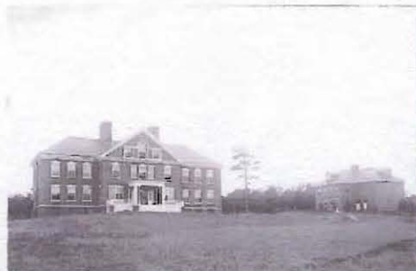
Administration Building at MCTS
