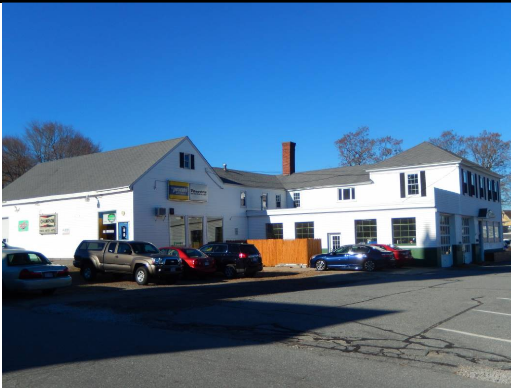
9 Princeton Street, facing northwest. May 2016.
